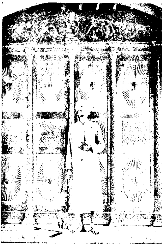
Carpenter and his work.
